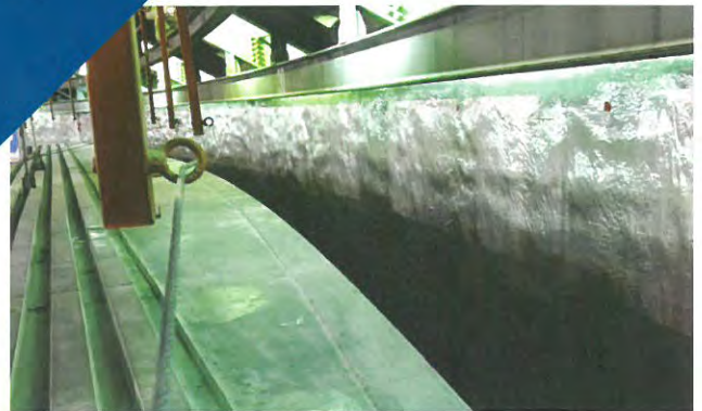
UNDER-GROUND TANK, INSIDE
